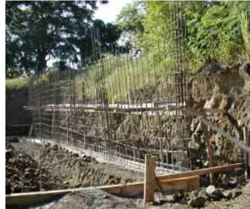
Back retaining wall of school
