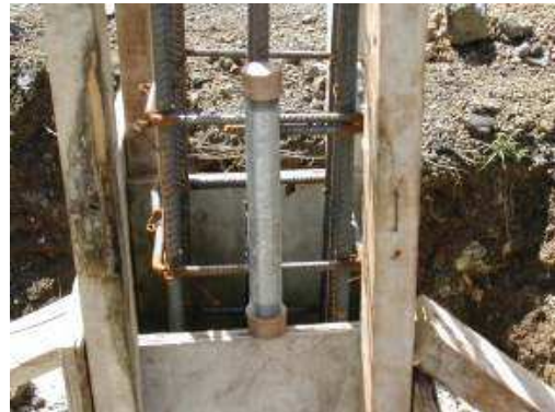
Putting our prayer tube in the foundation
