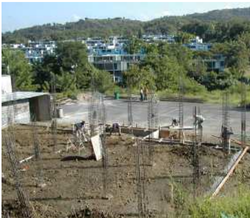
Looking down on the site from road
