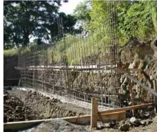
Back retaining wall of school
